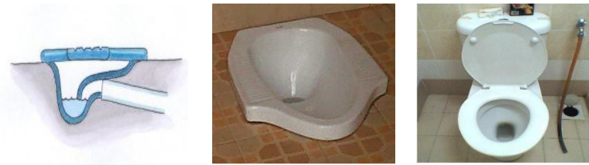
Toilets with a goose-neck with U-shaped pipe
